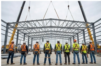
Team of 10 Workers Positioning Large Truss in PPE.
