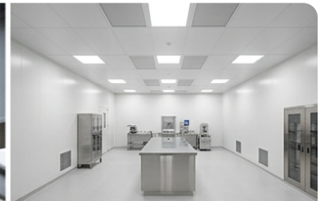
Completed Clean Room with Smooth Panels and LED Lighting.
