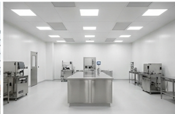
Completed Clean Room with Smooth Panels and LED Lighting.
