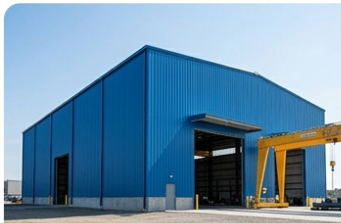
Erected Blue PEB Building with Operational Gantry Crane.
