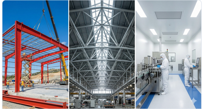
Grand architectural truss & clean space designs
