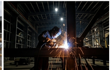
Night Shot of Structural Welding and Sparks.
