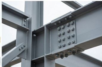
Close-up of Clean, Bolted Moment Connection.
