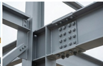
Close-up of Clean, Bolted Moment Connection.
