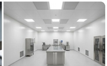
Completed Clean Room with Smooth Panels and LED Lighting.
