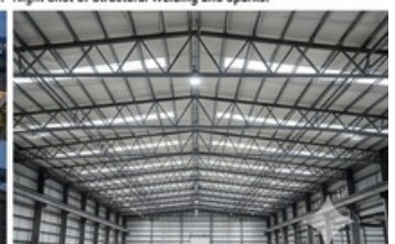
Intricate Open-Web Truss Roof System in Fabrication Hall.
