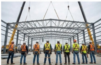
Team of 10 Workers Positioning Large Truss in PPE.
