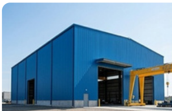
Erected Blue PEB Building with Operational Gantry Crane.
