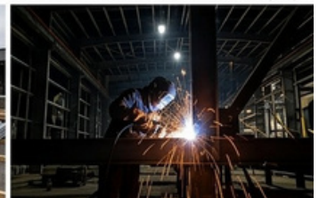
Night Shot of Structural Welding and Sparks.
