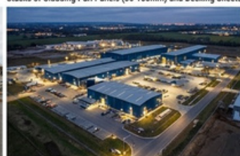
Sprawling Modern Industrial Manufacturing Plant and Steel Structure at Twilight.
